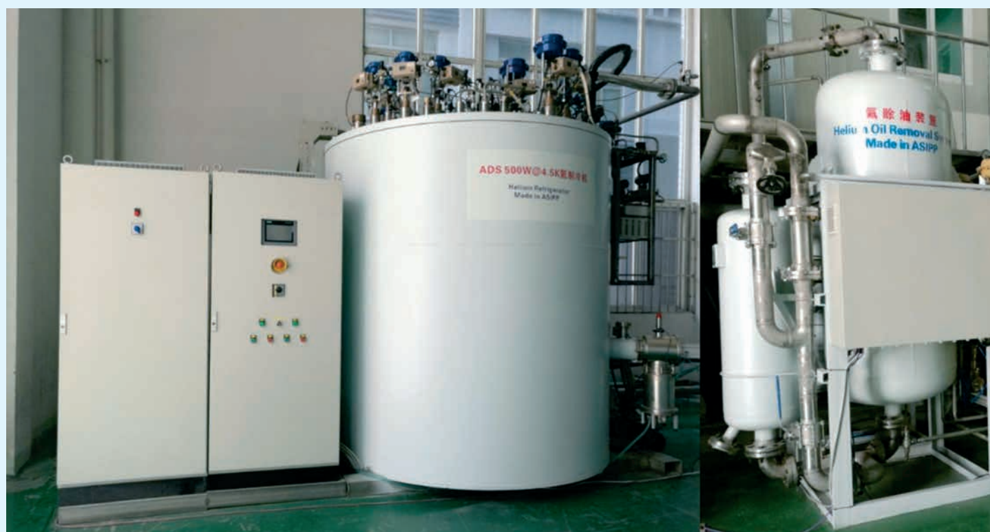
500W@4.5K helium refrigerator/liquefier
