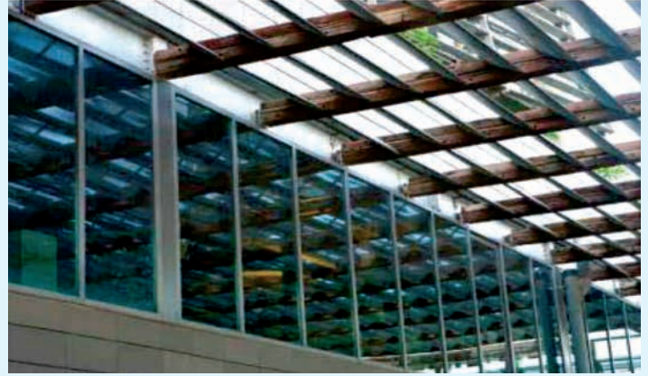
Photo 2: Shading devices installed on façade for controlling day-lighting and glare in indoor spaces.
