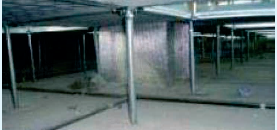
Photo 5: Photograph taken of the void space (below raised false floor to indicate floor insulation and UFDV).
